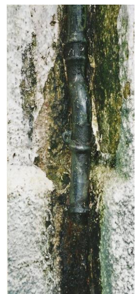
Figure 3: Broken Drain
