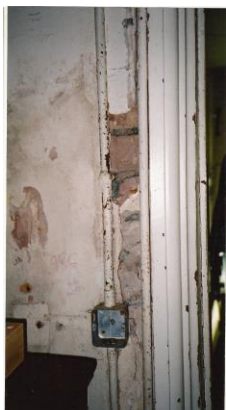
Figure 2: Water ingress
